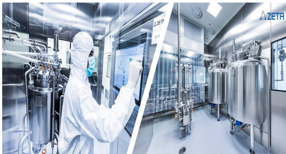
Advanced cleanroom design: software-controlled HVAC Source: web
