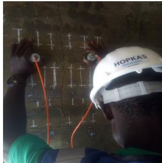
Figure 8: Field SHM in progress (2017)
