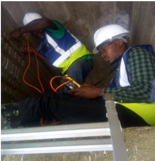
Figure 7: Field SHM in progress (2017)
