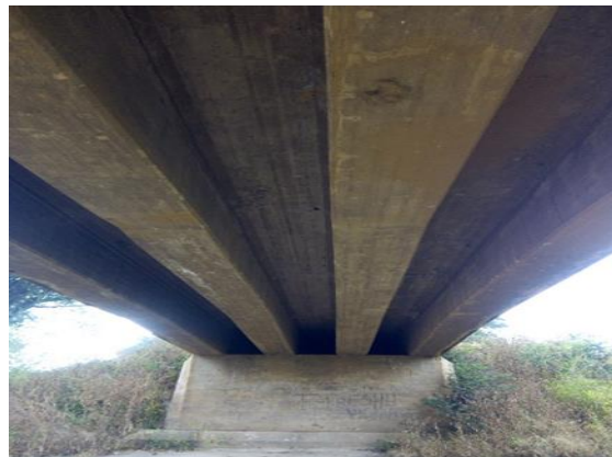
Figure 2: Beam-Slab Deck for Nansenga Bridge
