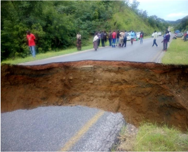
Figure 1: Sinazeze- Maamba Road (Source: Mwebantu Media)
