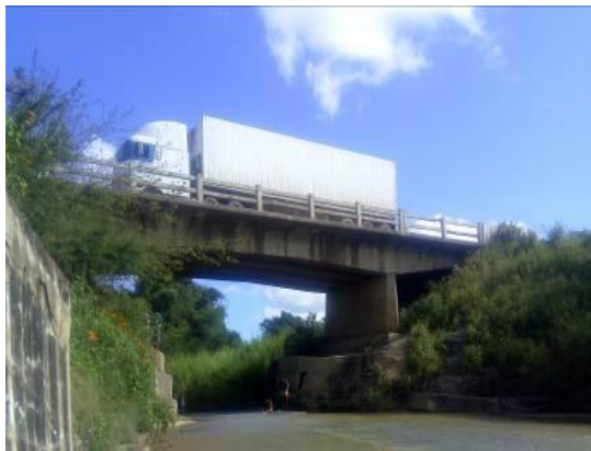
Figure 1: Side view of Nansenga Bridge
