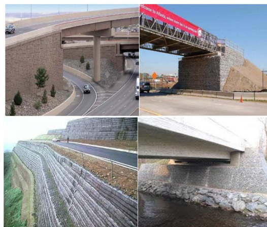
Figure 3: Applications of MSEW (Reinforced Earth Company, 2011).
