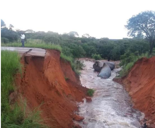
Figures 2a and 2b: Bridge crossings for the Lifune (left) and Msuzi (right) rivers washed away during the 2018-2019 rainy season.
