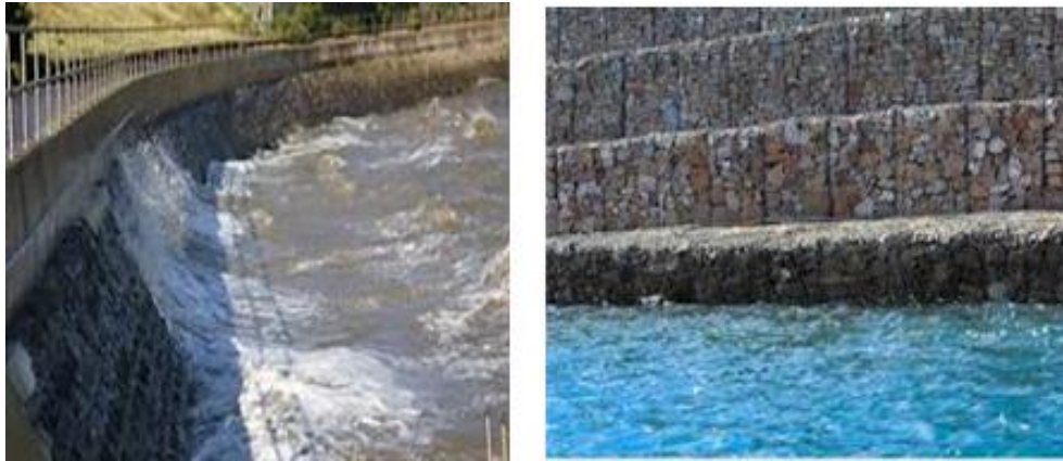
Figure 5: Gabions used for coastal defence (Maccaferri, 2010)
