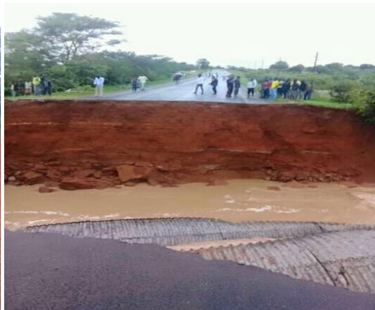
Figures 2a and 2b: Bridge crossings for the Lifune (left) and Msuzi (right) rivers washed away during the 2018-2019 rainy season.
