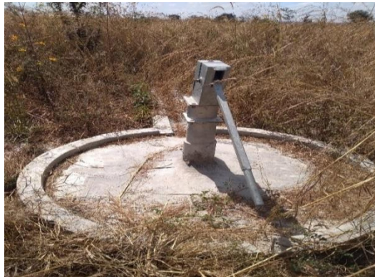
Figure 4: Dried up newly installed borehole in one of the resettlement lands
