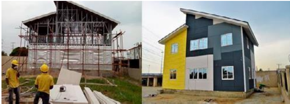
Figure 7. DCT office building at Chevron Lekki, Lagos Source; Cromrite 2020
